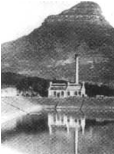
Molteno – Cape Town's first Power Station
